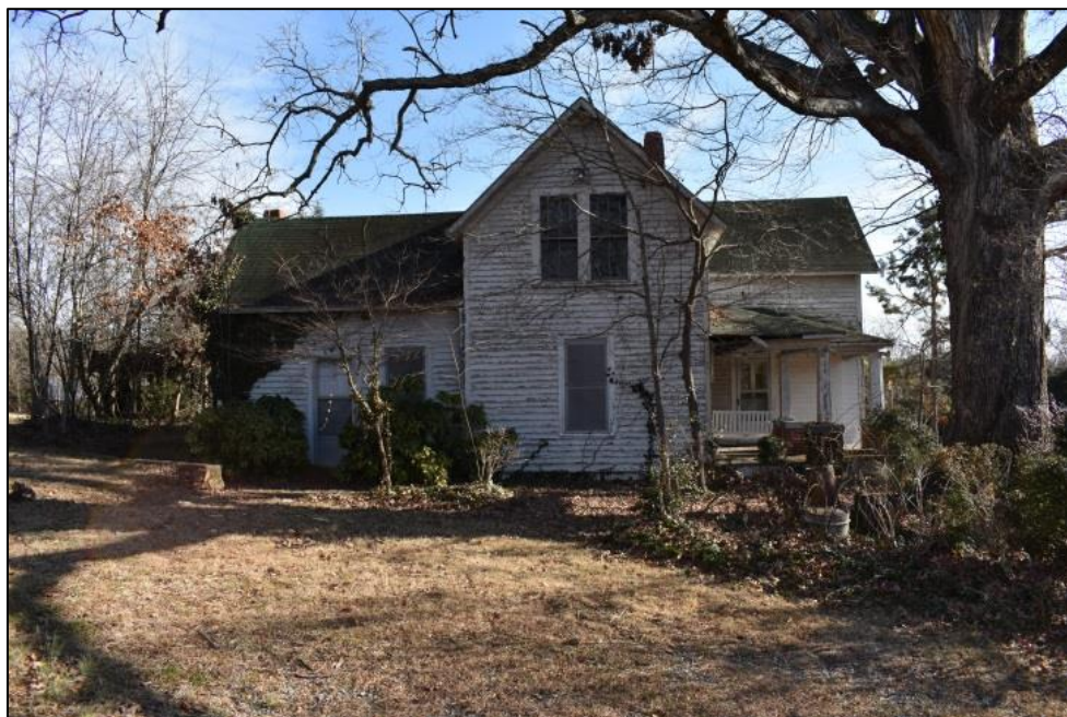
Figure 6: View of Stirewalt House's (west) side elevation with L-shaped main block at right and ell at left.
