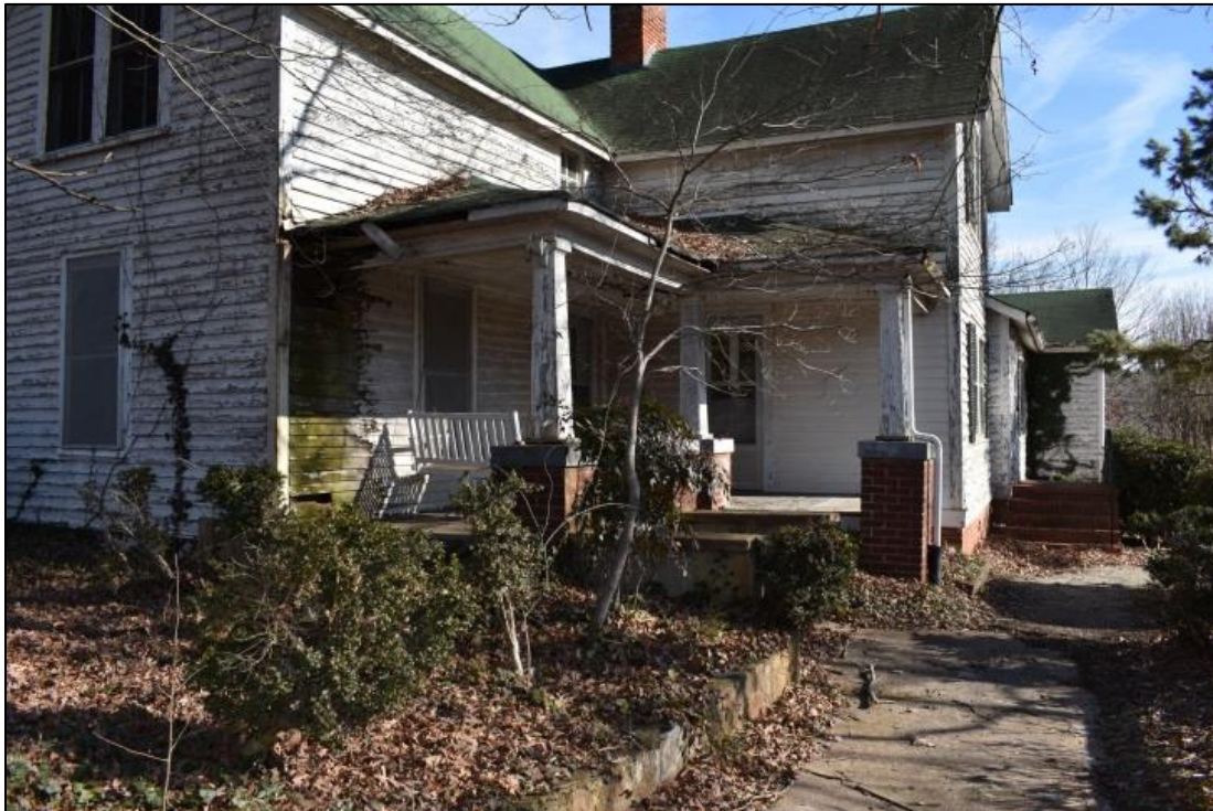
Figure 11: Detail of front porch (southwestern corner).
