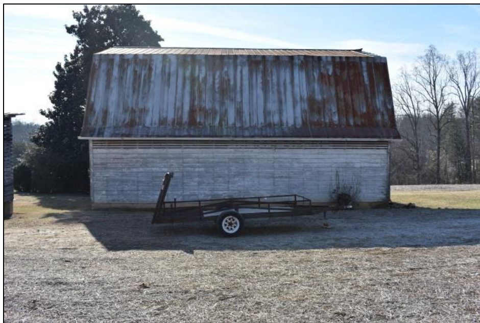
Figure 28: View of northern elevation of barn.
