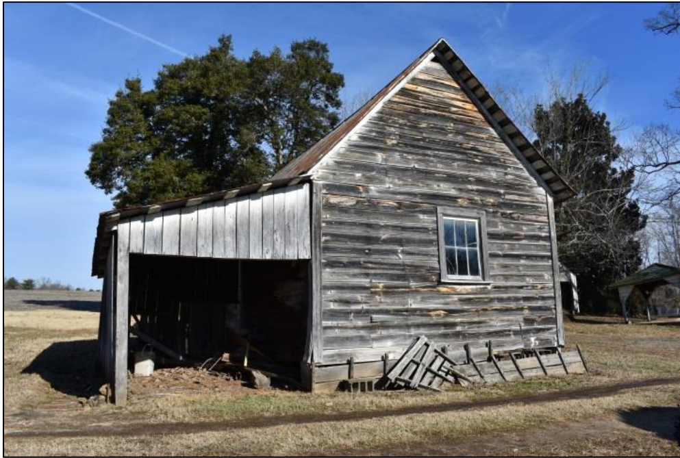
Figure 25: View of southern elevation of workshop.
