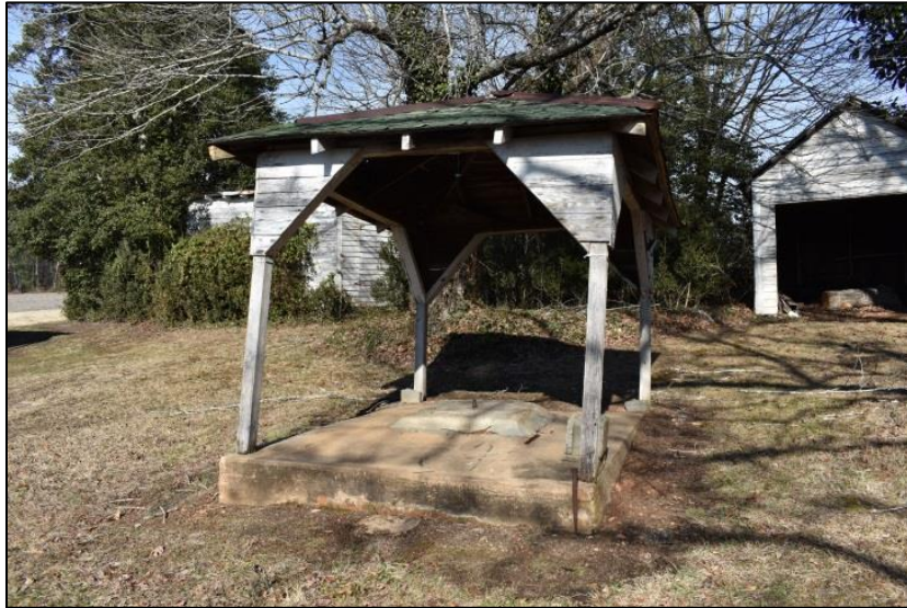
Figure 21: View of well house looking to the north.
