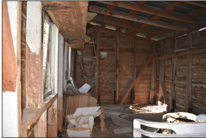
Figure 23: View of interior of west shed, looking to west.
