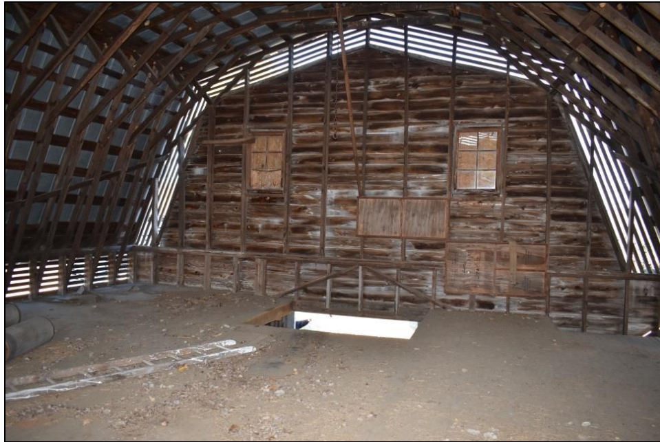
Figure 31: Interior view of second floor, looking to east.
