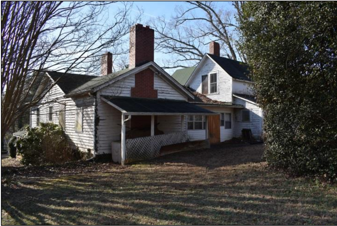
Figure 10: View of northeastern corner of rear elevation.
