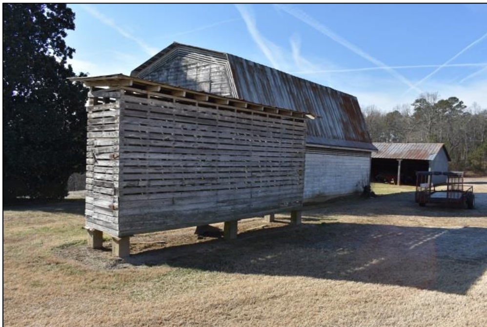
Figure 26: View of rear (northern elevation) of corn crib.
