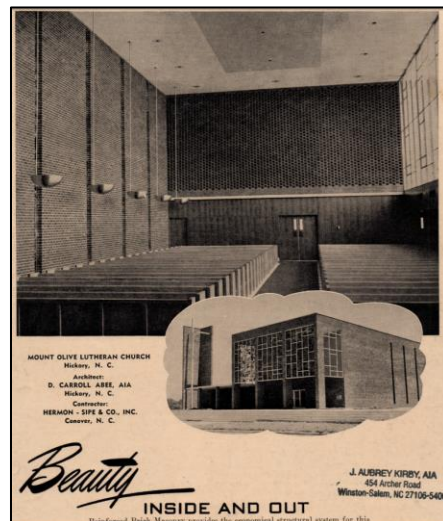
Figure 63: Images of Mt. Olive Lutheran Church lauding its use of reinforced brick masonry, walls with vertical slits glazed with stained glass, and “open-textured brick organ screen” (Southern Architect 1959)
