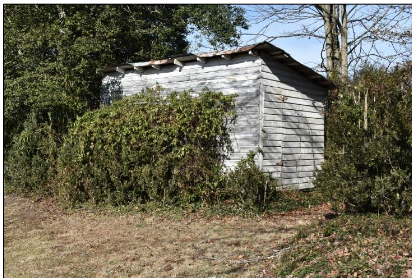
Figure 22: View of southeastern corner of west shed.
