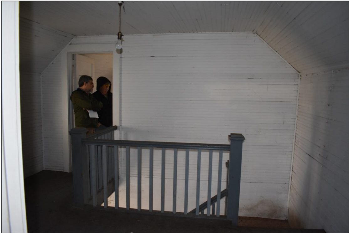
Figure 17: View of second floor stairwell in original block, looking to west.
