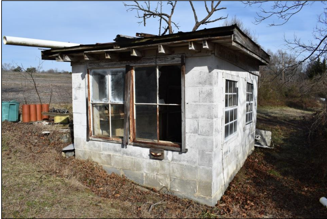
Figure 38: View of concrete shed, looking to northeast.
