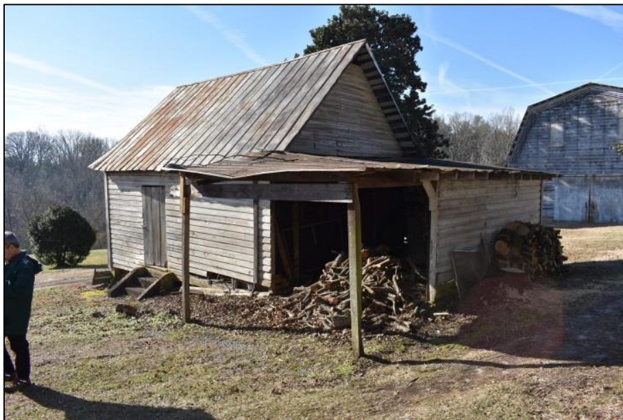
Figure 24: View of northeastern corner of workshop.
