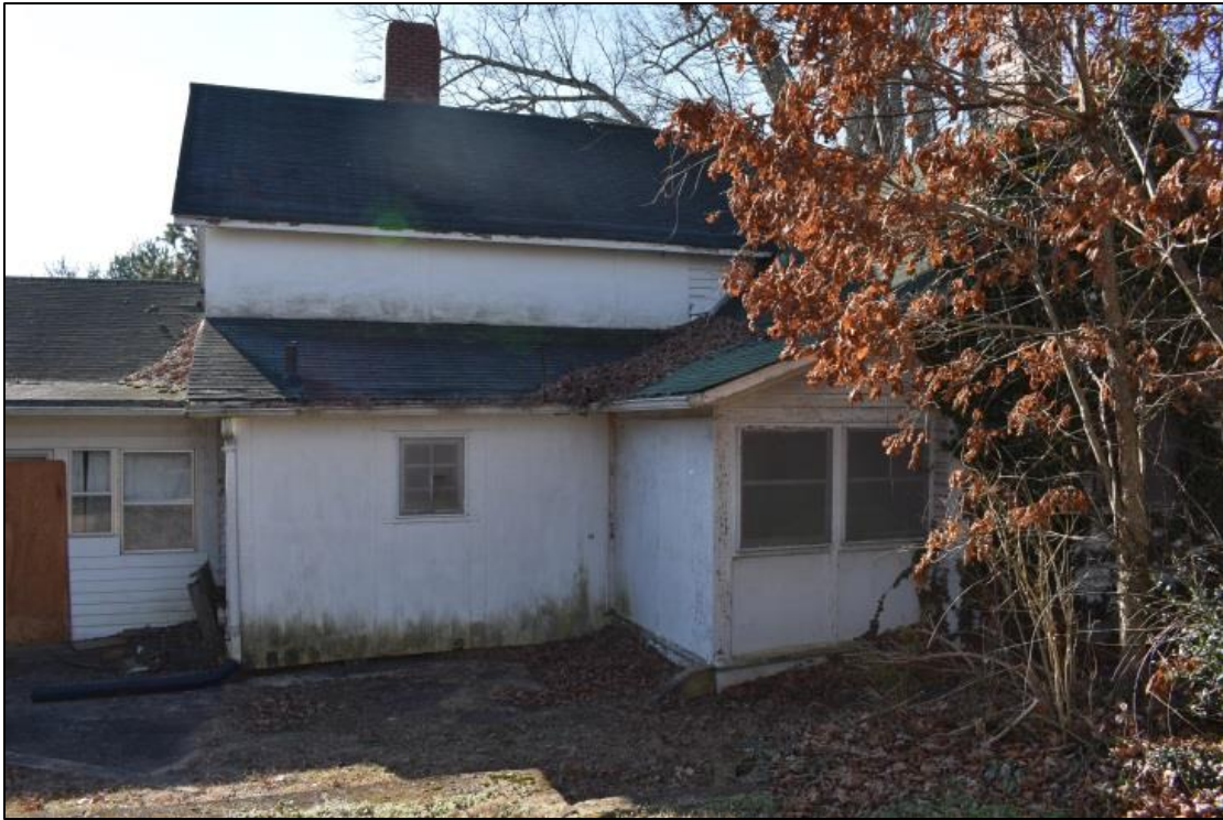
Figure 12: View of northwestern corner of rear elevation; note partial re-siding.
