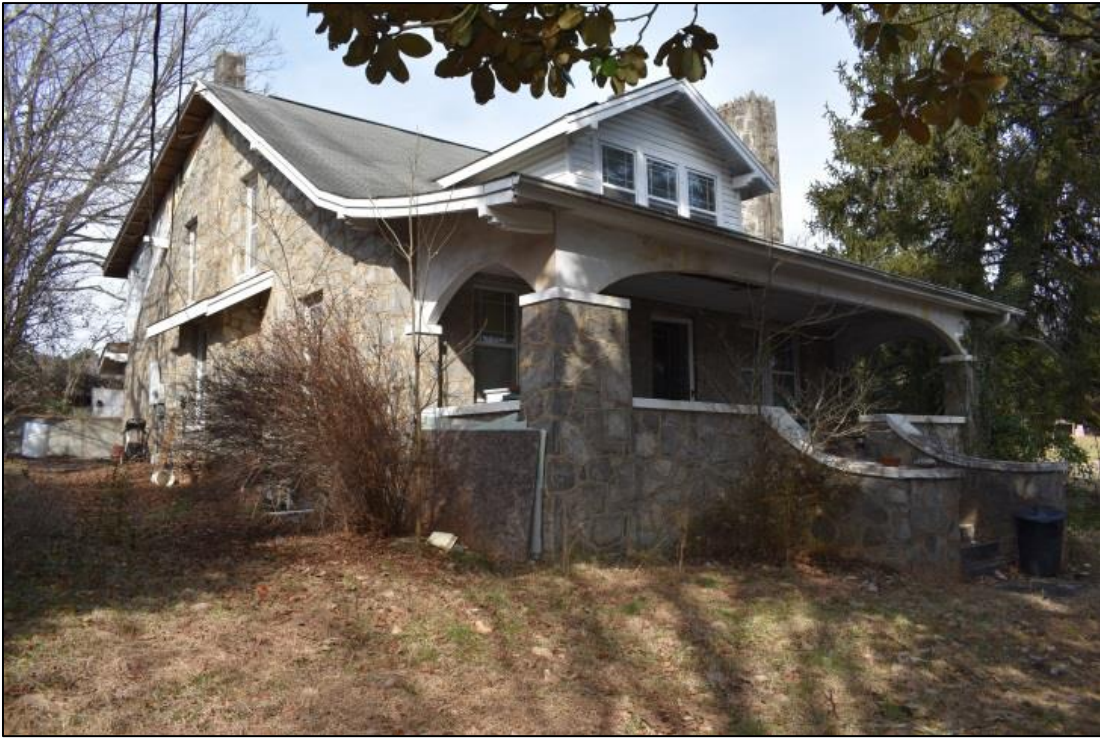
Figure 36: View of southwestern corner of Ledford House.
