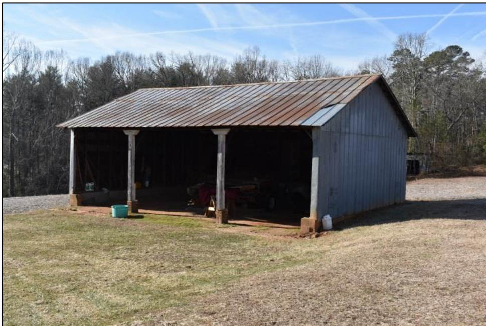
Figure 32: View of northeast corner of tractor shed.
