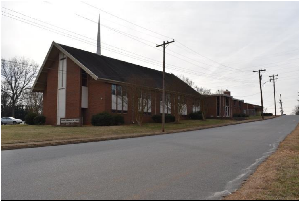
Figure 51: View of northeastern corner of church with education wing to rear.
