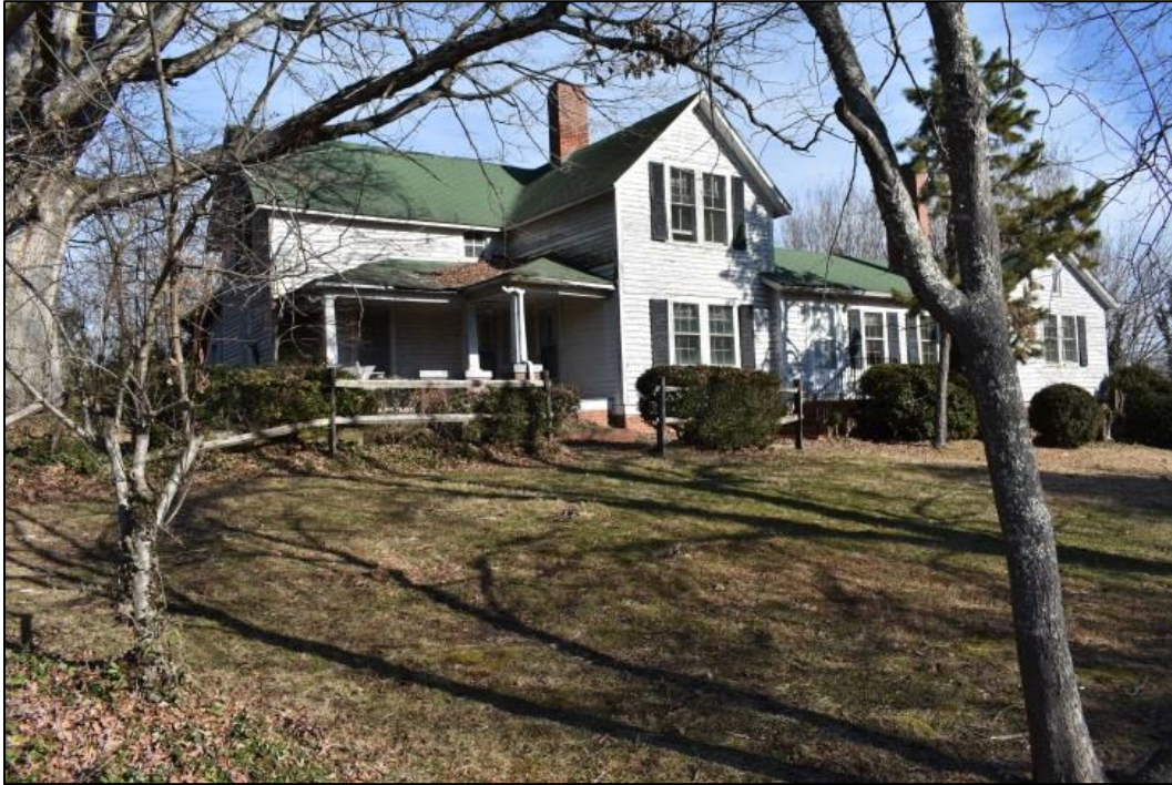
Figure 7: View of front elevation (southwestern corner).
