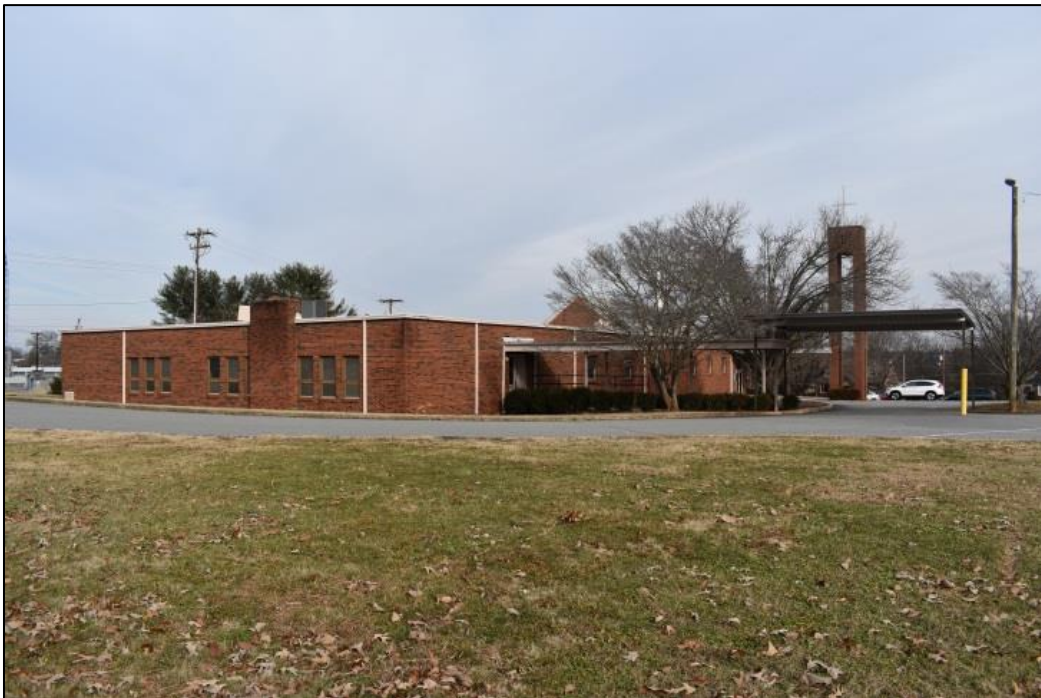
Figure 52: View of northwestern corner of education wing with rear gable of church rising at the center.
