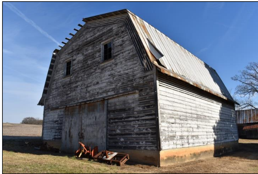
Figure 29: View of northeast corner.
