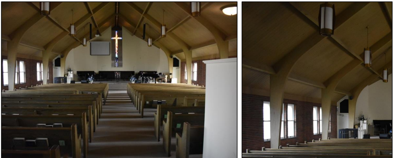
Figure 54: View of interior of sanctuary, looking north, with roof detail at right.
