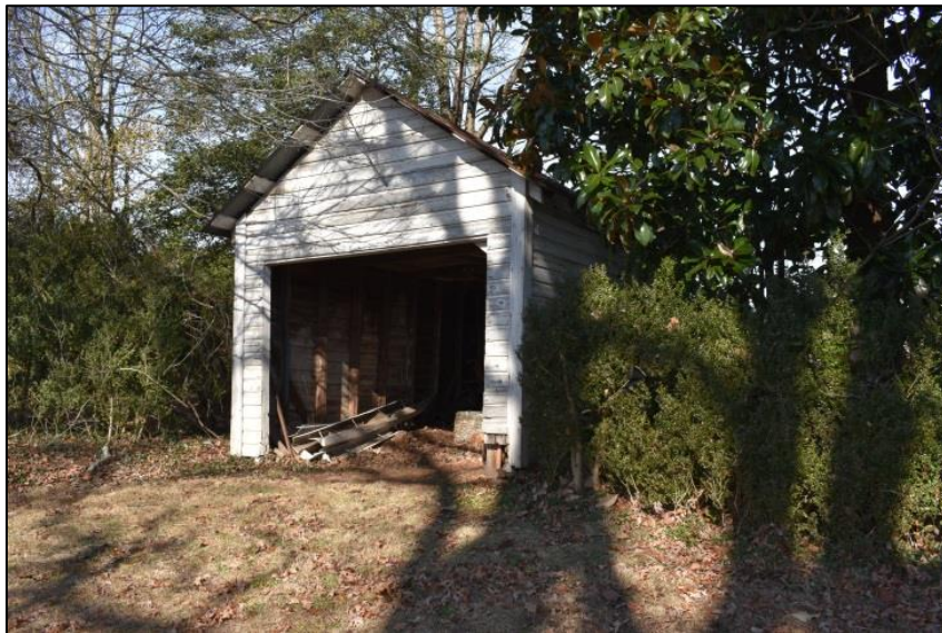
Figure 20: View of southeastern corner of garage.
