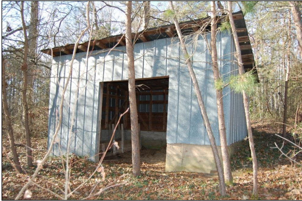
Figure 33: View of eastern elevation of birthing shed.
